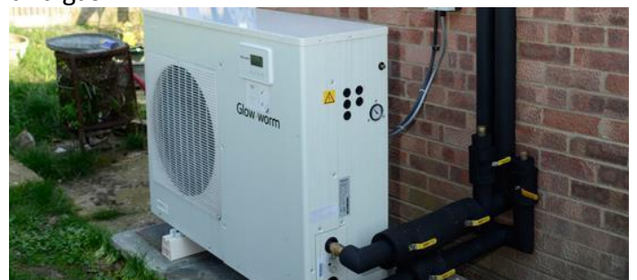
A typical air source heat pump
