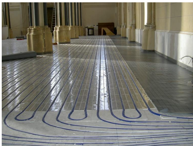
Heating pipes being built into a raised church floor
