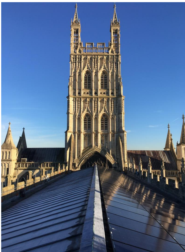
Solar panels on Gloucester Cathedral. The 150 solar PV panels will generate 29,000 kW of energy a year, enough to power seven semi-detached houses or make 250,000 cups of tea per year. Energy costs will be reduced by 25 percent, saving £190,000 over the next twenty five years.
