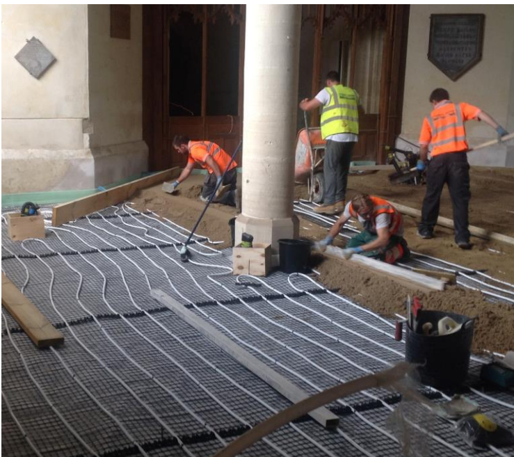
Installation of a typical underfloor heating system
